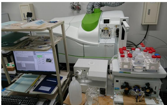
Picture 3. NexION 350S inductively coupled plasma mass spectrometer installed in the Fukushima Prefecture's laboratory
